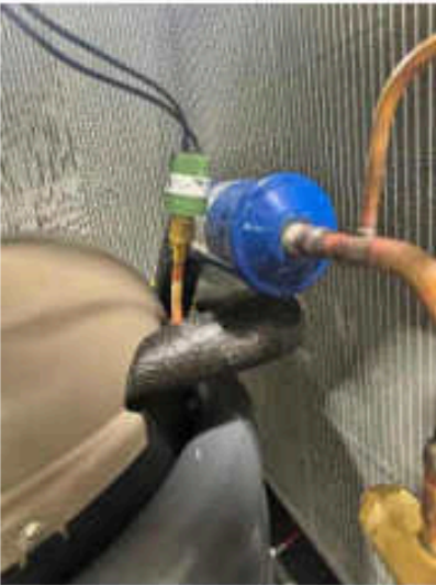
THE HIGH-PRESSURE SWITCH HAS BLACK WIRE LEADS.
