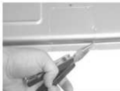
FIGURE 11 REMOVING CONDENSATE KNOCKOUT
