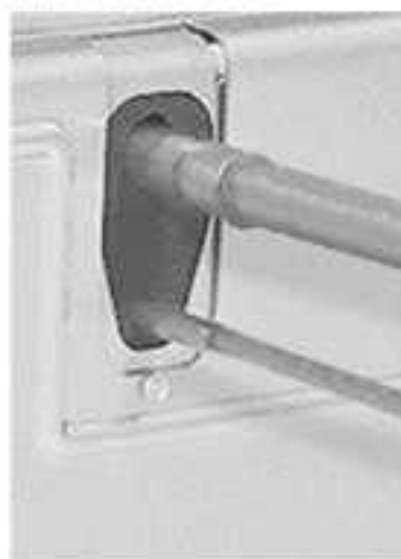
FIGURE 9 COMPLETED REFRIGERANT CONNECTION ASSEMBLY
