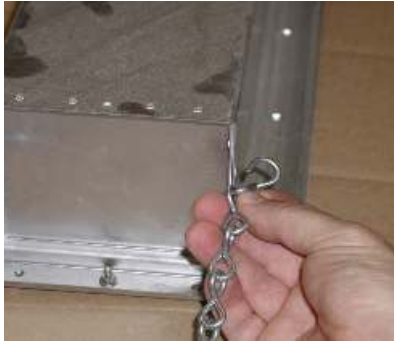
FIGURE 6: ATTACH SUSPENSION HARDWARE
