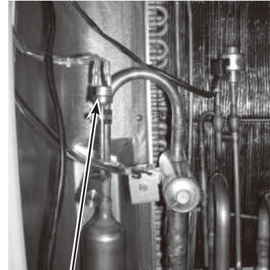
High pressure switch (63H)
